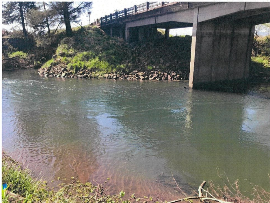
Photo 4: View of the south bank at bridge, with existing riprap armor.
