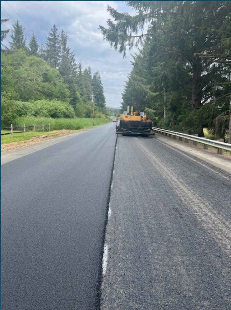
PAVING SANDLAKE ROAD
