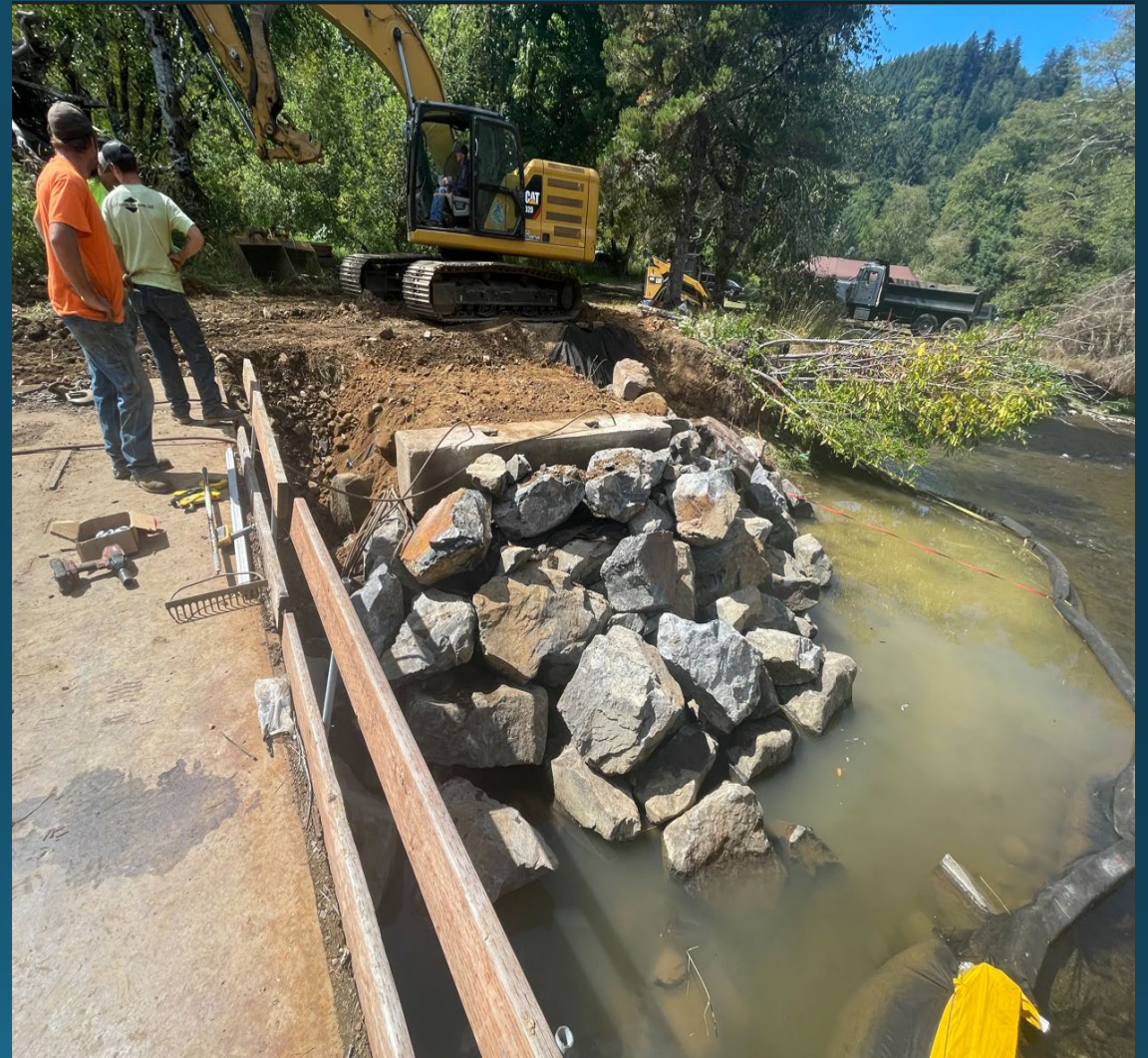
BIG TROUT BRIDGE—SEPTEMBER 2023 DEADMAN SYSTEM INSTALLATION
