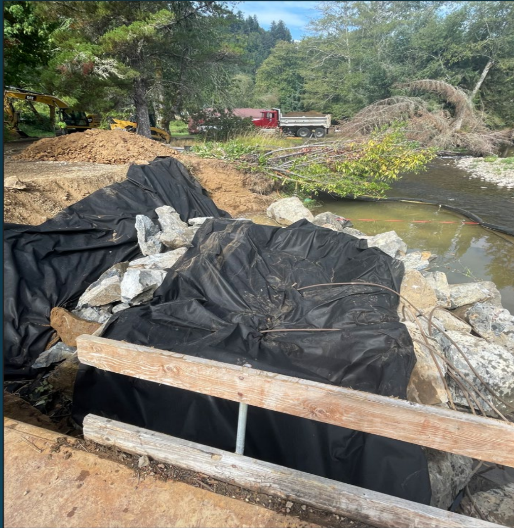
BIG TROUT BRIDGE—SEPTEMBER 2023 DEADMAN SYSTEM INSTALLATION
