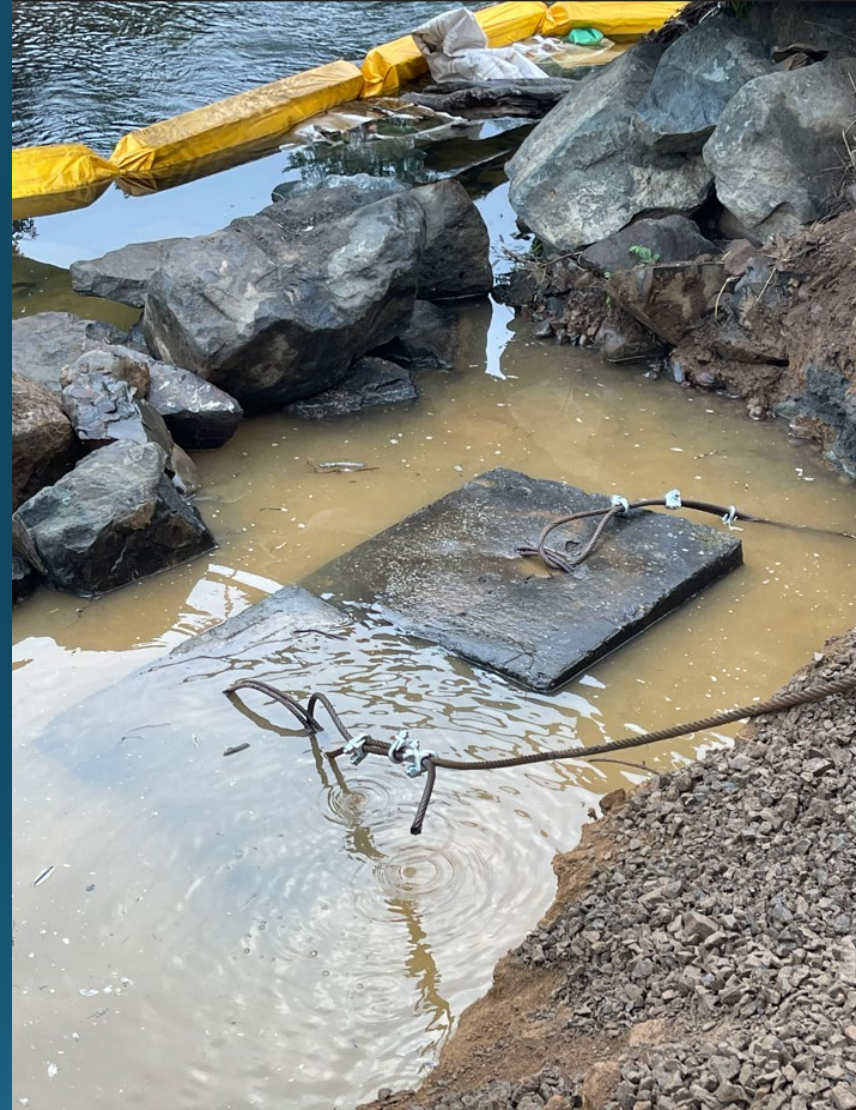
BIG TROUT BRIDGE—SEPTEMBER 2023 DEADMAN SYSTEM INSTALLATION
