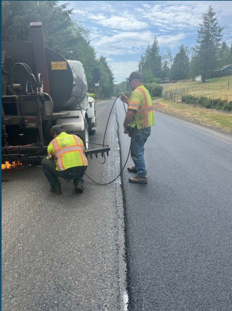
PAVING SANDLAKE ROAD
