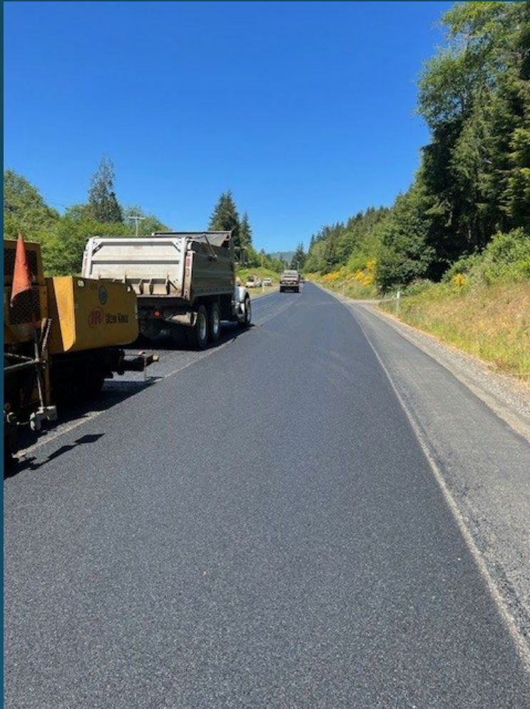
PAVING SANDLAKE ROAD
