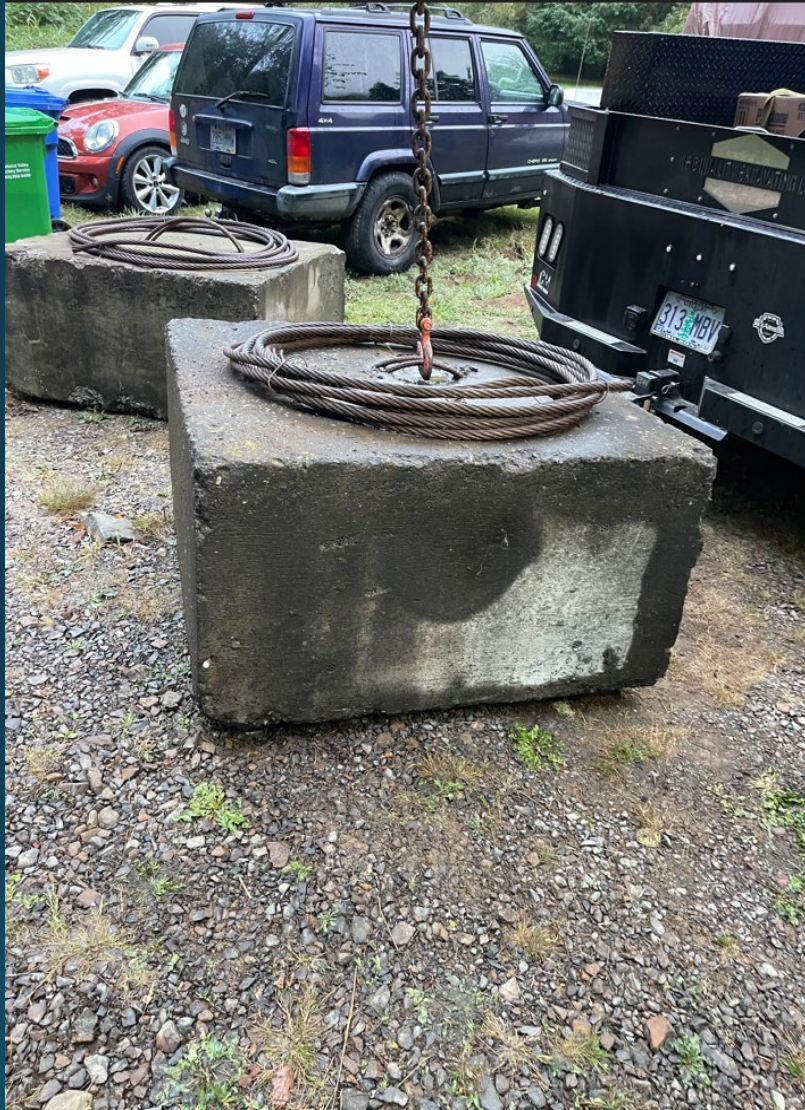
BIG TROUT BRIDGE—SEPTEMBER 2023 DEADMAN SYSTEM INSTALLATION
